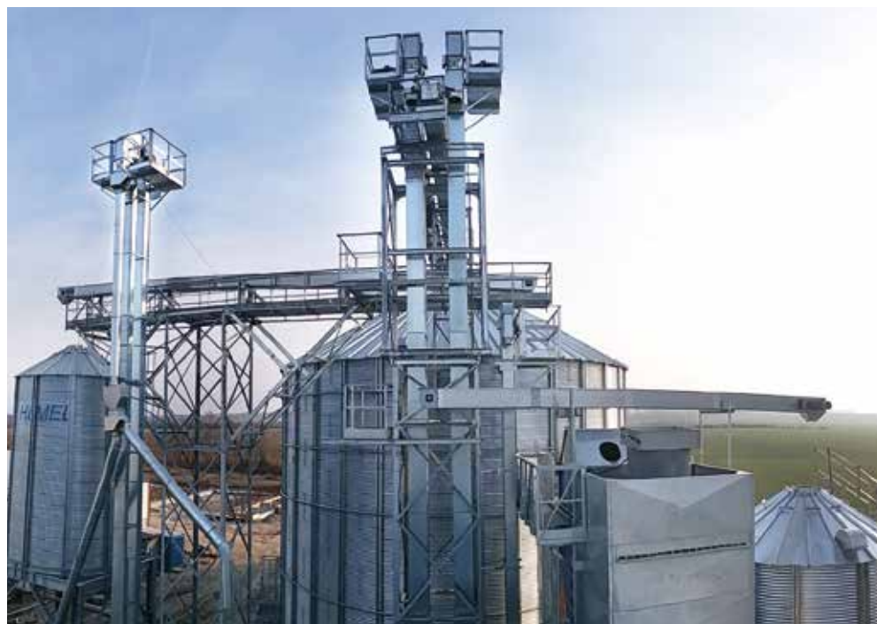
HIMEL Becherelevatoren in Getreideanlage
